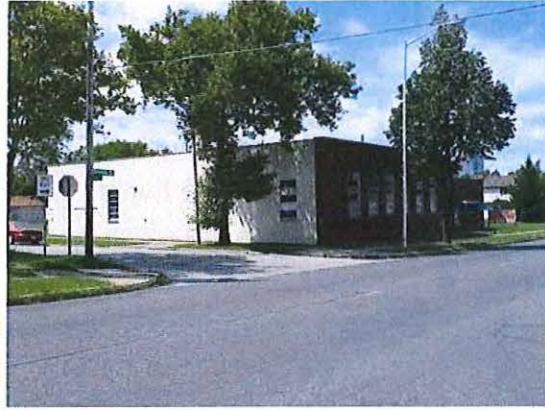
2050 Lafayette Street Doolittle Electric 02-12-11-431-019.000-074
