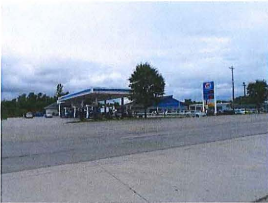
2420 W. Jefferson Blvd. Marathon Gas Station 02-12-09-226-002.000-074
