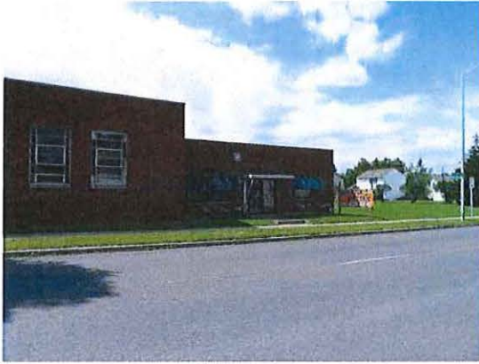
2050 Lafayette Street Doolittle Electric 02-12-11-431-019.000-074
