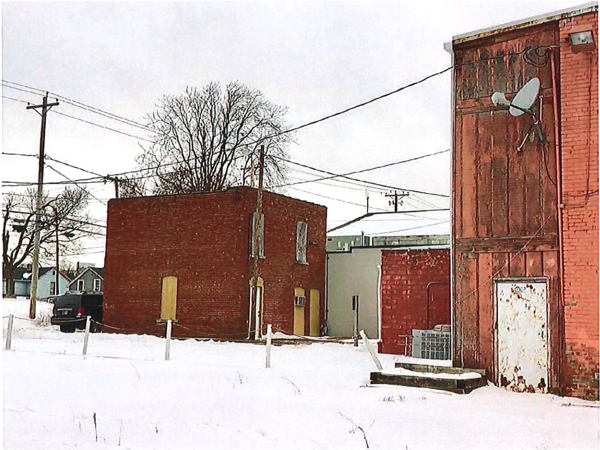
View of Zuber Carriage House behind 2020 Fairfield.
