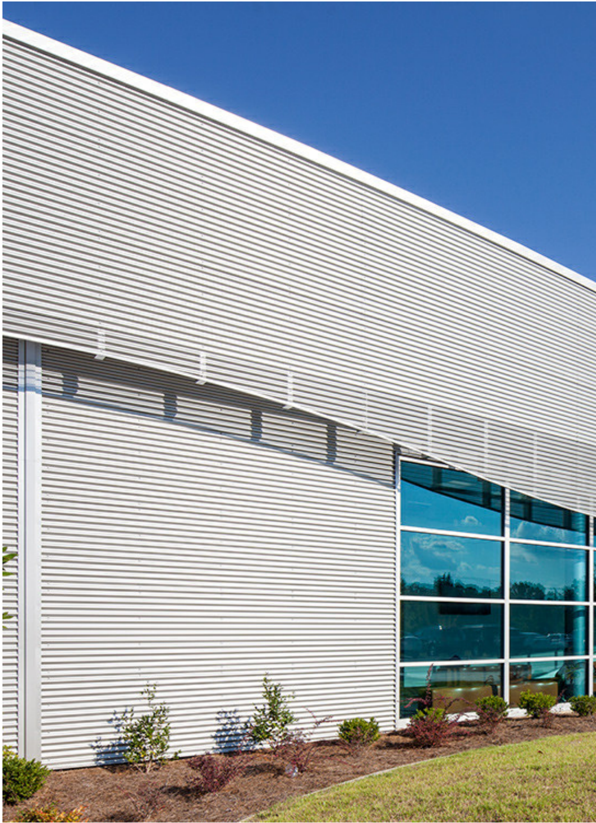
EXAMPLE: CORRUGATED ARCHITECTURAL METAL PANEL PROPOSED FOR THE GREY AREAS OF THE BUILDING
