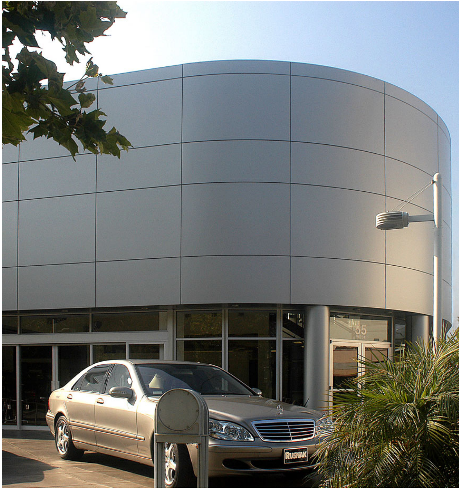
EXAMPLE: ACM (ARCHITECTURAL COMPOSITE METAL PANEL) PROPOSED FOR THE BLACK AREAS OF THE BUILDING
