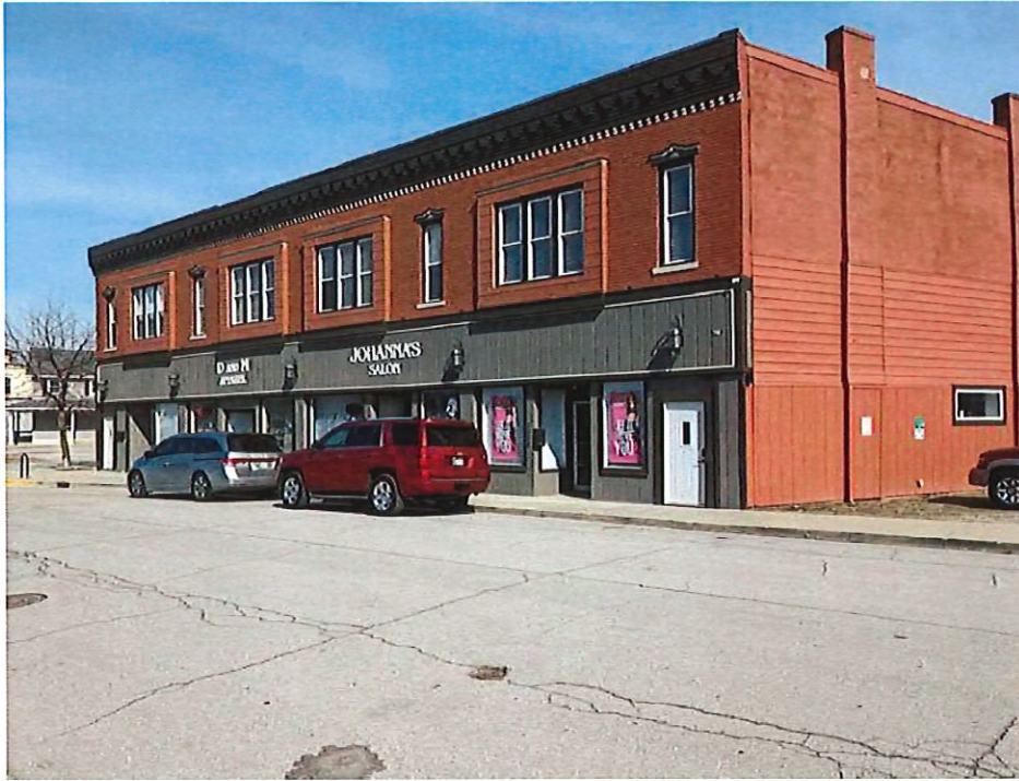
Façade and South Elevation
