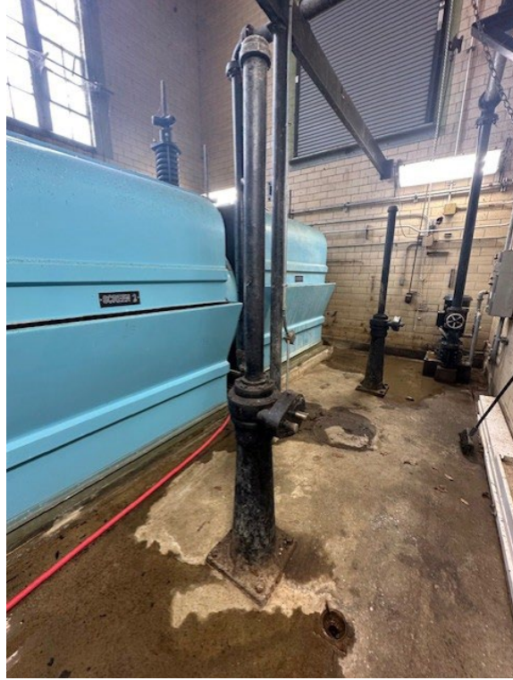
Figure 13 (Left): Sluice Gate #1 on Pump Side for Screen Channel #1
