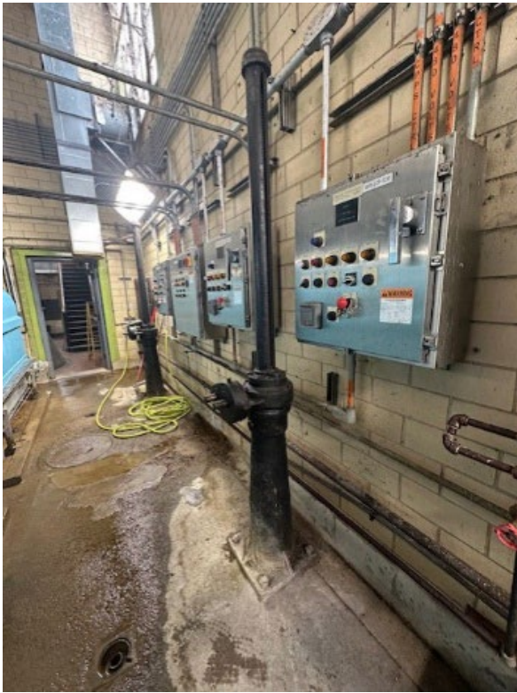
Figure 17 (Left): Sluice Gate #2 on River Side for Screen Channel #2 Figure 18 (Right): Sluice Gate #3 on River Side for Screen Channel #3
