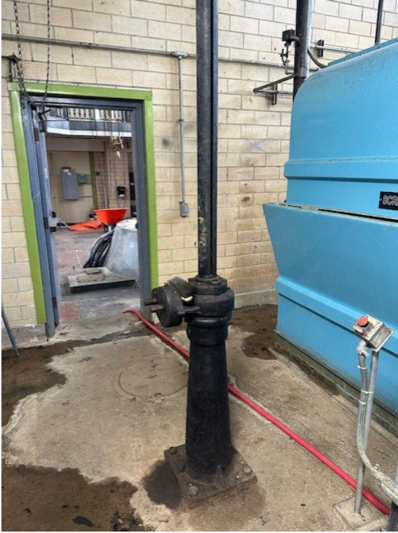
Figure 13 (Left): Sluice Gate #1 on Pump Side for Screen Channel #1
