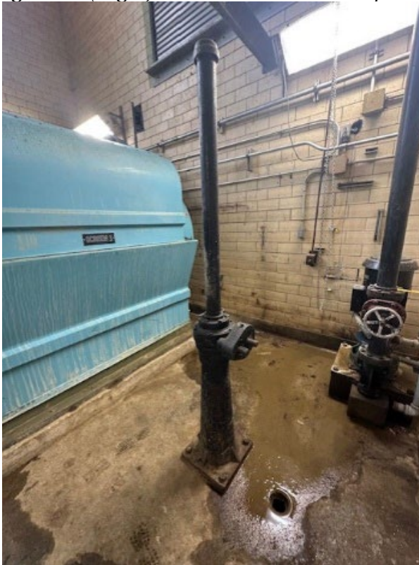
Figure 15 (Left): Sluice Gate #3 on Pump Side for Screen Channel #3
