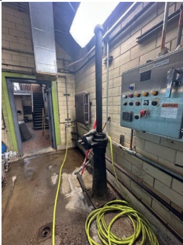
Figure 15 (Left): Sluice Gate #3 on Pump Side for Screen Channel #3
